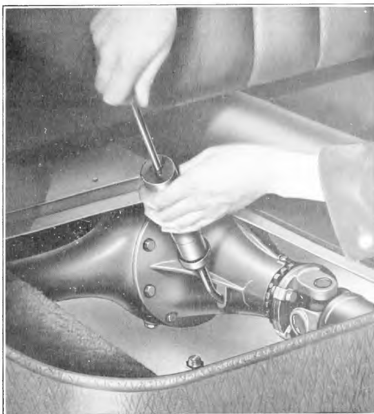
Fig. 33 Topping up Rear Axle
